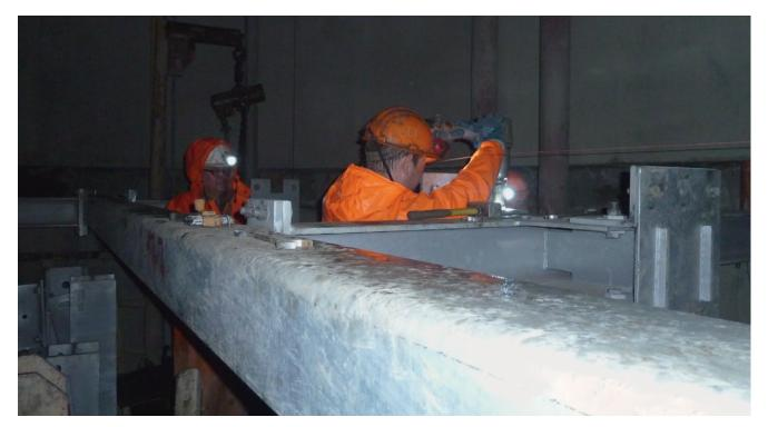
Shaft buntons are installed in parallel with shaft sinking in WS-10
