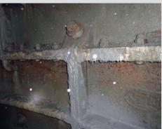
Leakage of grouting material between tubbings
