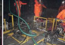
Pic. above left: Injection mounting for the sealing material "NOH20"
