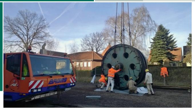
Demounting of the old hoisting engine drum
