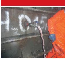
Pic. left: Shaft sinkers while grouting work inside the foreshaft
