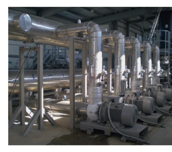
Centrifugal pump for circulating refrigerant or heating medium
