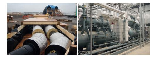
Pic. left: Encased brine pipes toward the shaft
