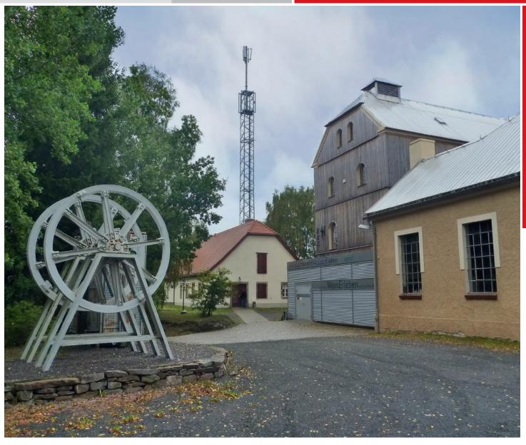
,Three Brothers Shaft' with cobbing table, mine shaft building and machine building
