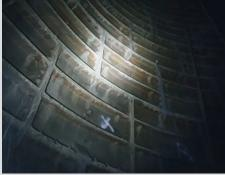
The grouting material take effect, the tubbing surfaces are drying
