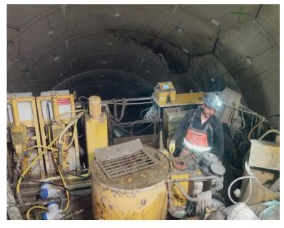
Grouting material being injected through the concrete tubbings in the inclined shaft
