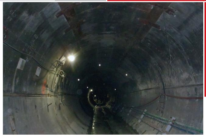
The primary MDS-tunnel with concrete-segment lining
