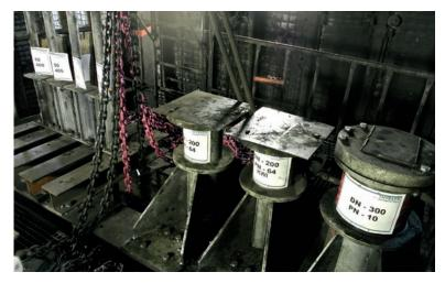
Support structures of supply circuits
