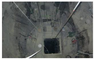
slipform, engineered shoring was required to establish a base for the concrete-steel transition embedded.
