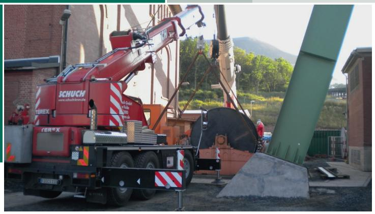
Tramming and sighting of 30t-hoist with truck-mounted crane, shaft Neuhof
