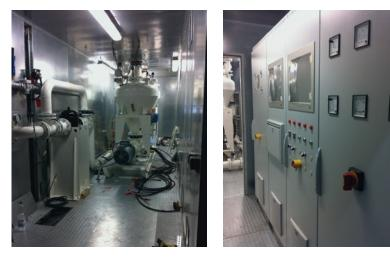
Tandem-transmitter-station with associated control system
