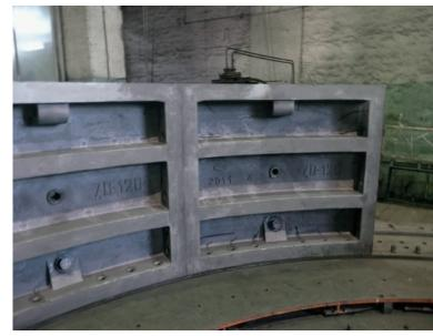
Test assembly of the cast iron tubbing segment at the surface.
