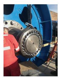
Mounting of the bearing on the main shaft
