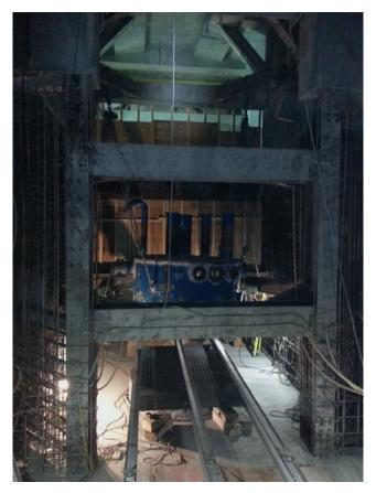
Construction of Upper RWT Using Engineered Skid Beams Over Transition Cone; Looking West
