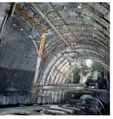
weldmesh lagging, the steel arch supports were set in place right along the roadway and immediately backfilled with concrete.
