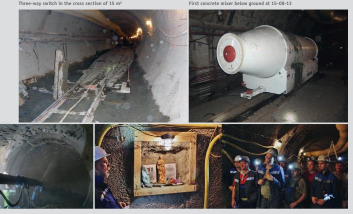
Shot crete manipulator MEYCO Oruga with telescopic arm applicate the first support layer
