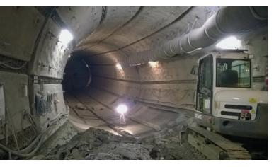
Transport roadway north, bottom excavation with excavator
