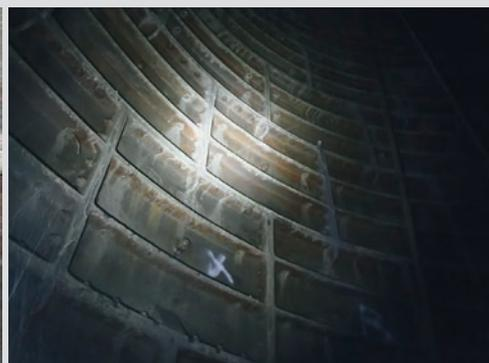
The grouting material take effect, the tubbing surfaces are drying
