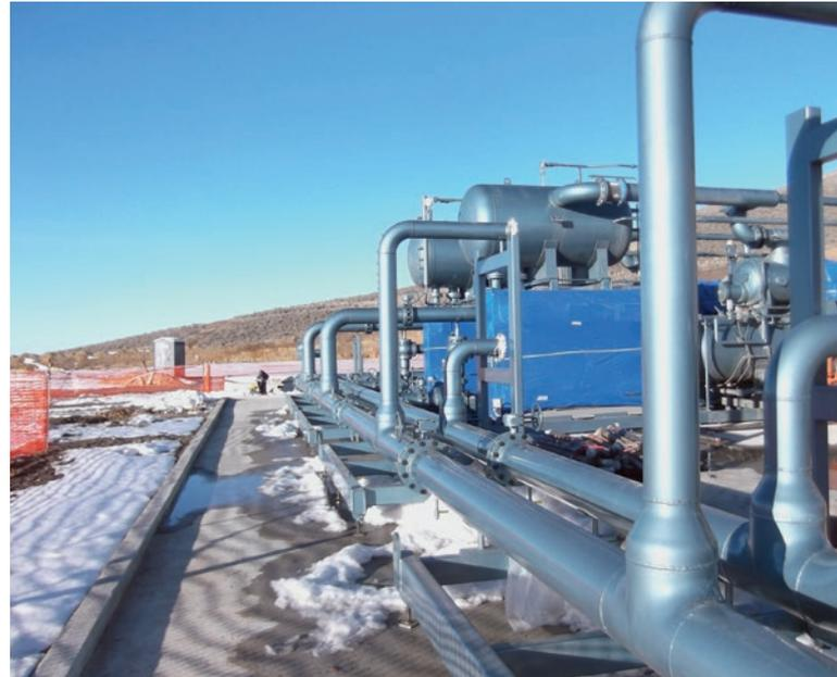
into a set of brine pumps which pumped brine to the shaft through a containment trench. The shaft site is quite small and fitting all of the required equipment close to the shaft proved challenging.
