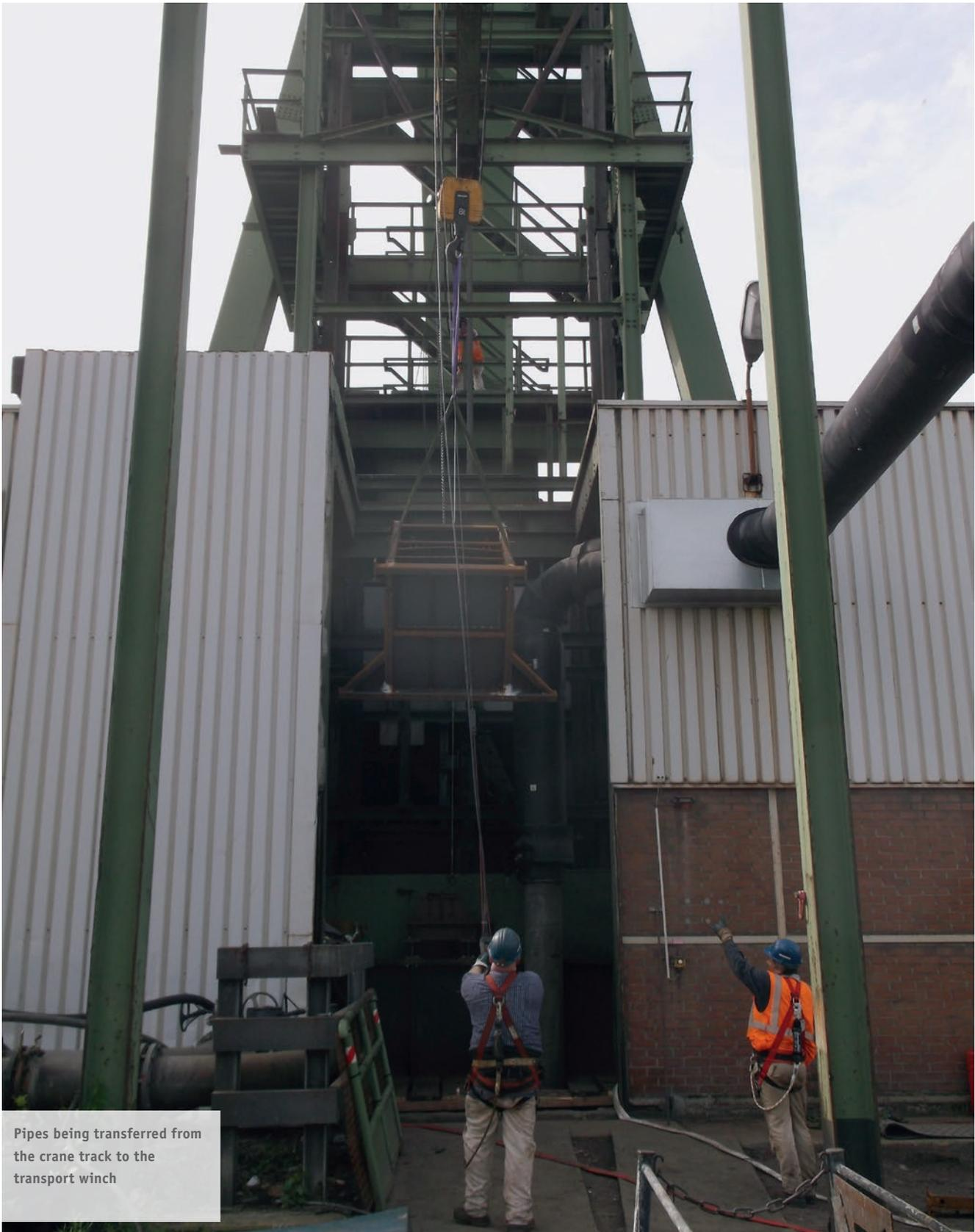
Pipes being transferred from the crane track to the transport winch
