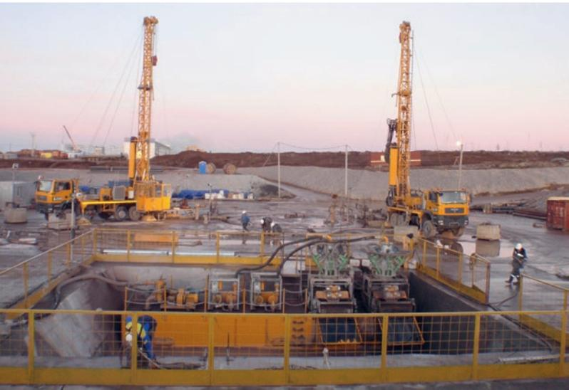
Freeze hole drilling, freezing and unfreezing in the Russian Federation
