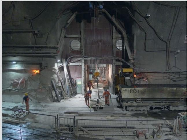
Pic. left: Transportation of heavy loads: lowering at shaft head
