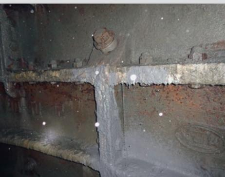
Leakage of grouting material between tubbings
