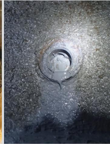
The grouting material is leaking out from an expansion hole
