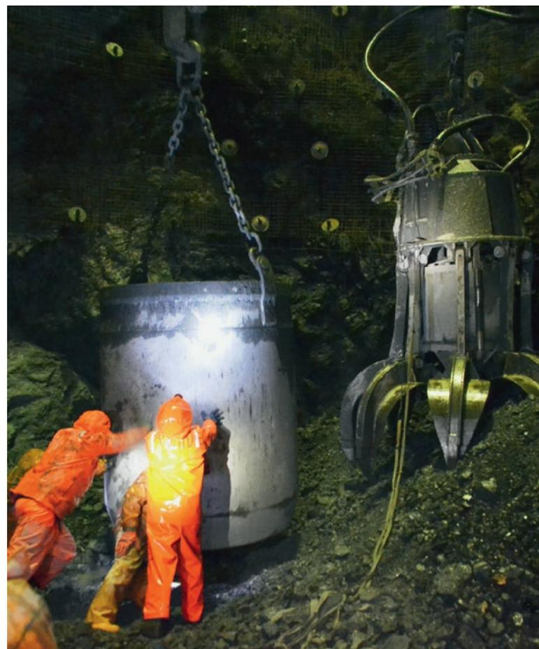
Loading sinking debris with the 1.2 m<sup>3</sup> grab and 5 m<sup>3</sup> bucket
