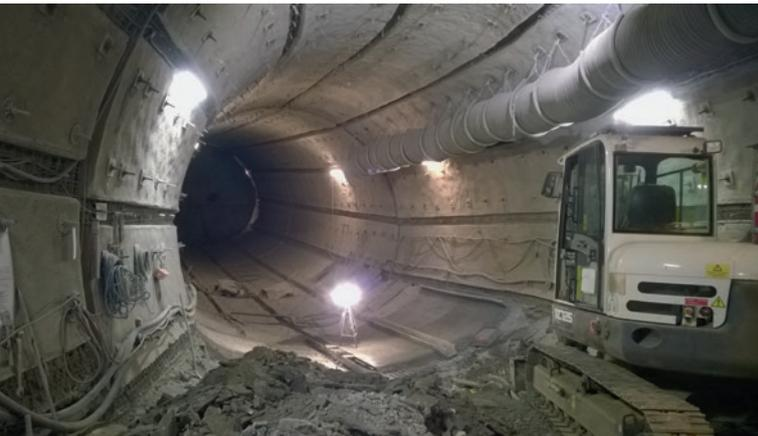
Transport roadway north, bottom excavation with excavator
