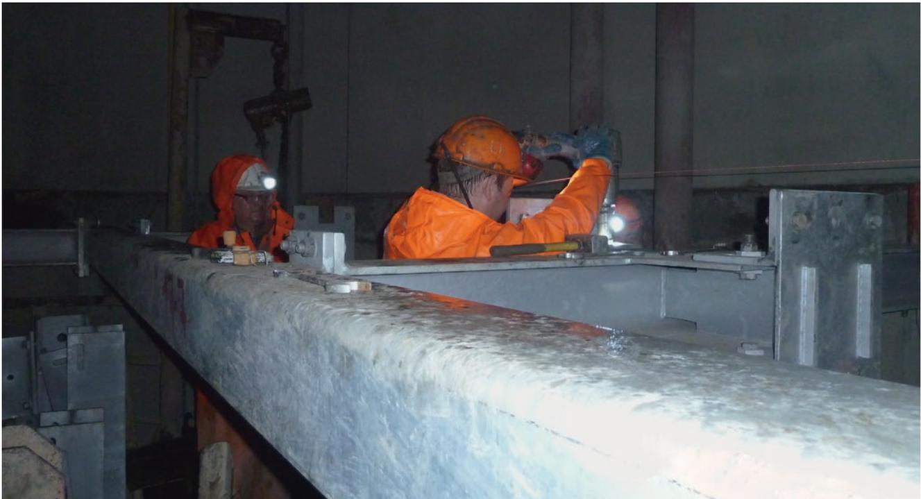
Shaft buntions are installed in parallel with shaft sinking in WS-10
