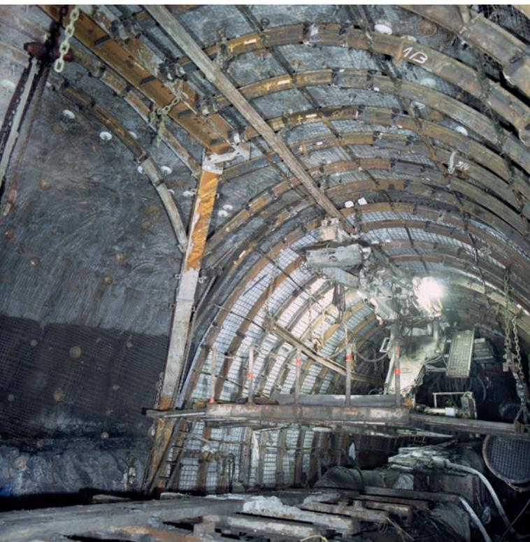
weldmesh lagging, the steel arch supports were set in place right along the roadway and immediately backfilled with concrete.
