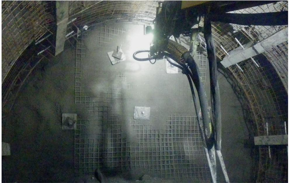
If the ground conditions worsen to a point where the open excavation (supported with hollow core dowels and shotcrete skim coat) is unsafe, the tunnels are advanced in a two-thirds, one third manner where the upper two thirds are always supported ahead of the excavation and shotcreting of the lower third, ensuring the workers are always under supported ground. Again, this methodology can also change as ground conditions change.
