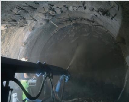
Shotcrete manipulator MEYCO Oruga with telescopic arm applicate the first support layer
