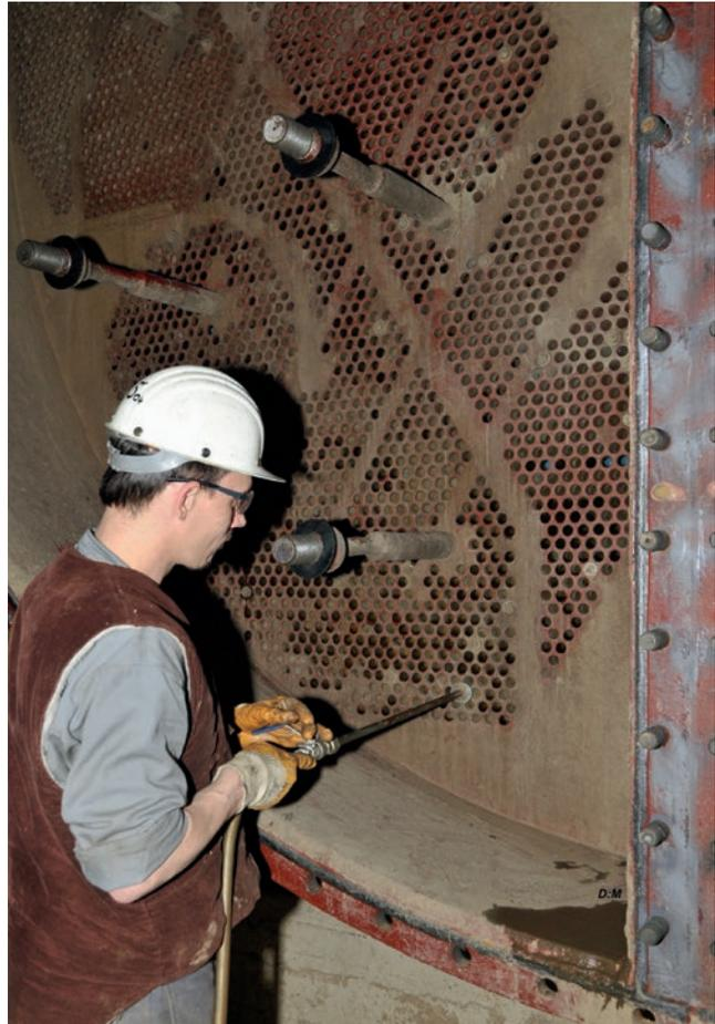
Pic. above: Revision works on a condenser in the Hermann Wenzel power plant of ThyssenKrupp AG, TKSE
