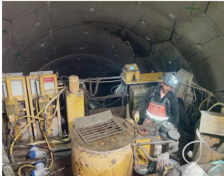
Grouting material being injected through the concrete tubbings in the inclined shaft
