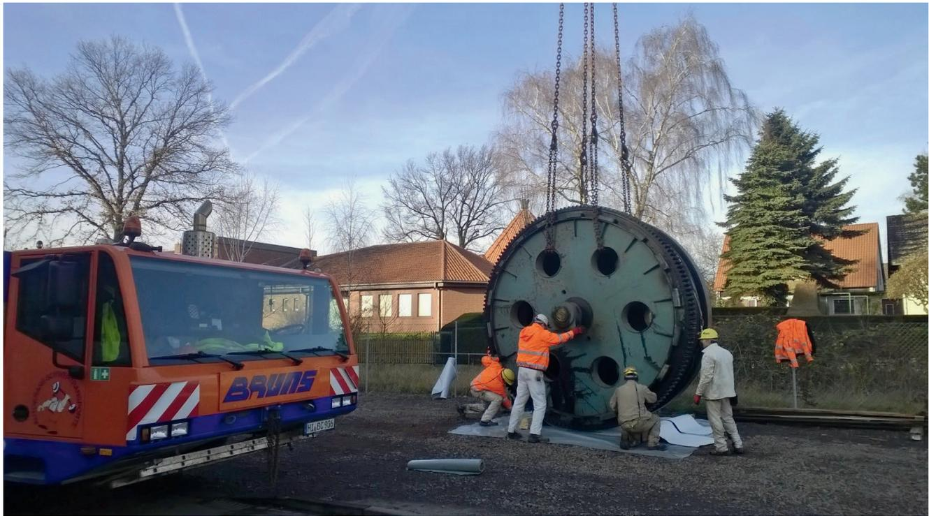
Demounting of the old hoisting engine drum
