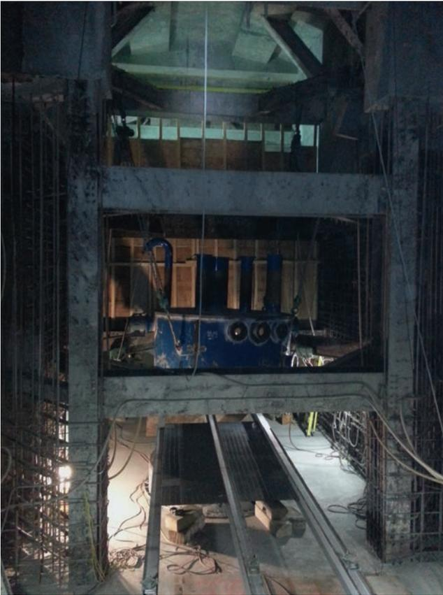
Construction of Upper RWT Using Engineered Skid Beams Over Transition Cone; Looking West
