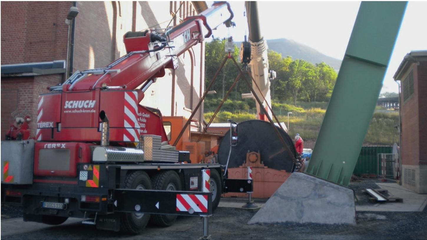
Tramming and sighting of 30t-hoist with truck-mounted crane, shaft Neuhof
