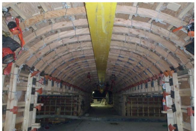
Concrete was poured in various stages to accommodate the elevated concrete floors. The floors were designed to rest on top of the concrete walls located in the center ROMS, making scheduling of concurrent construction activities more challenging. These intricate pours required engineered shoring as well as highly skilled forming and the strategic placement of critical embeds and anchor bolts.
