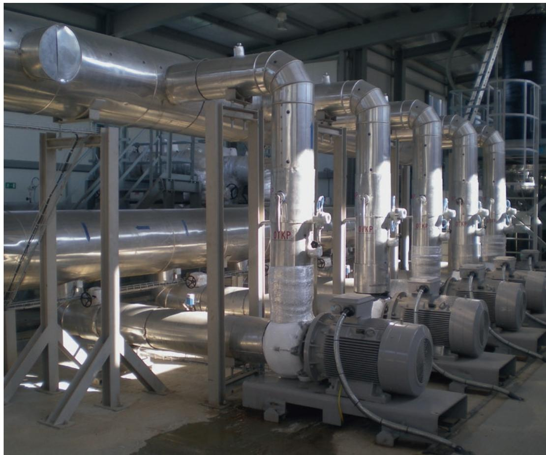
Centrifugal pump for circulating refrigerant or heating medium
