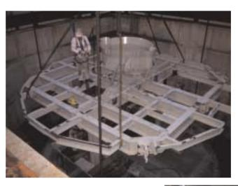
of the working platform was opened and the existing 3-deck conveyance removed section by section. The bottom deck was subsequently set on supports at the mouth of the shaft to act as an overhead screen during the headgear rebuilding phase.
