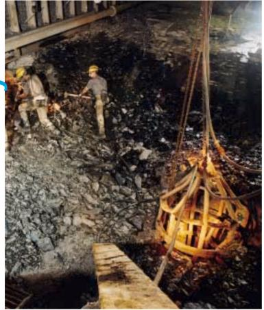
Over the next two years Deutsche Steinkohle's Ensdorf colliery plans to construct four coal bunkers in the Primsmulde production field so that the existing cost-intensive and uneffective coal conveyance circuit can be improved by a new product transport system. This coal bunker project will in conjunction with the Primsmulde ventilation shaft help safeguard the medium and long-term future of Ensdorf colliery.
