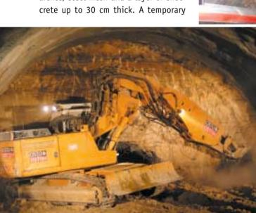
Tunnel excavator clearing the heading face (friable dolomite from the Upper Muschelkalk Series)
